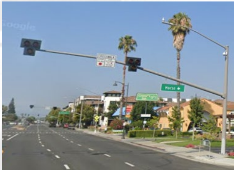
Ped Hybrid Beacon System
